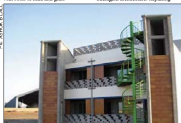
Cavities in the walls insulate an apartment in Bellary, Karnataka.
